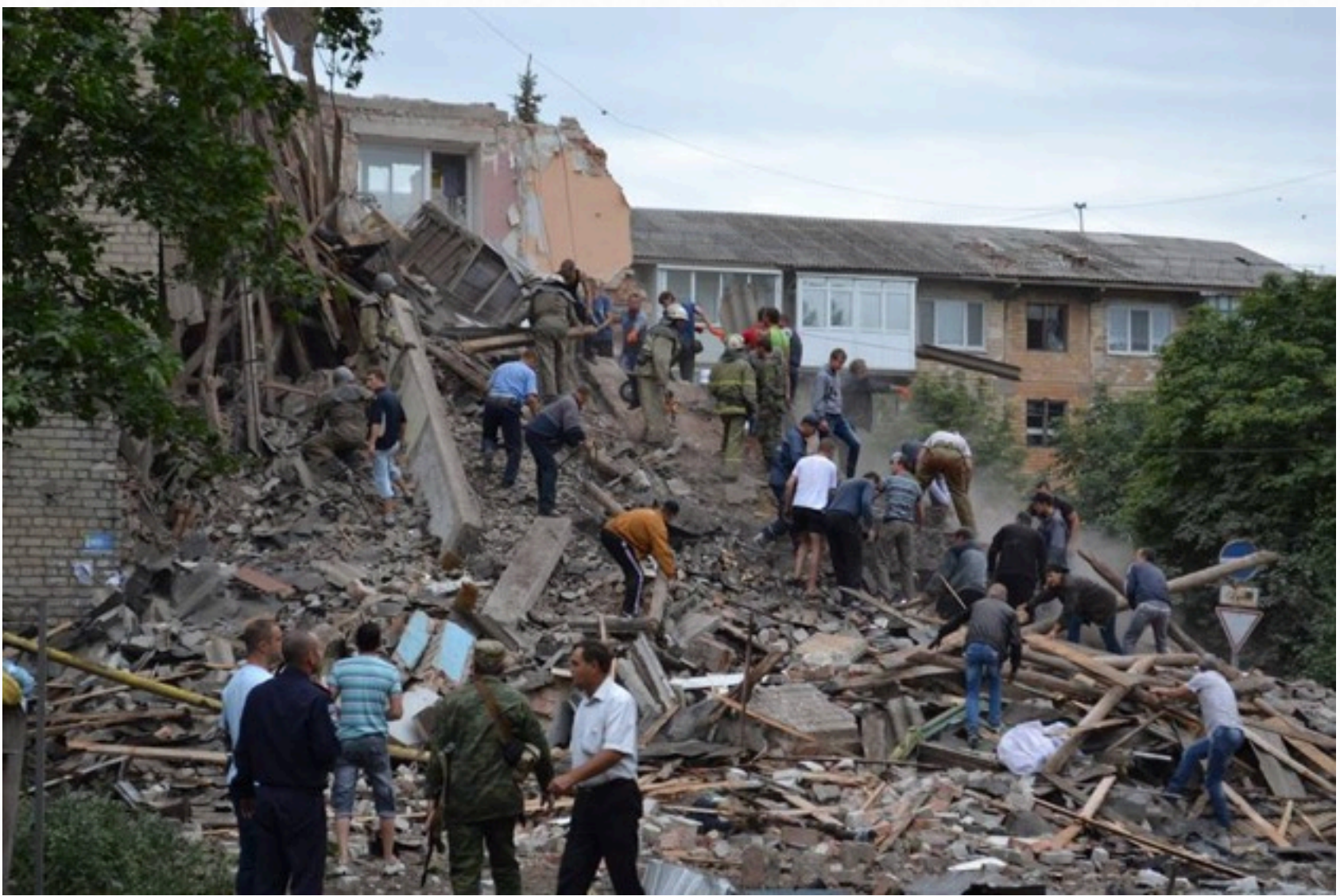
The aftermath of a Ukrainian air strike that hit an apartment building, leading to the deaths of eleven civilians
